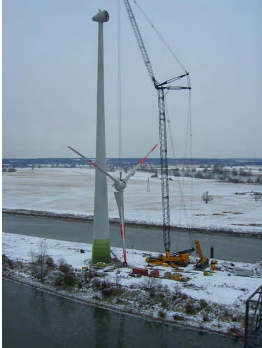
Figure 3.9: Erection of an Enercon E70-4 in Germany
