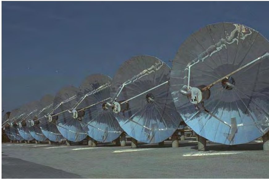
Figure 3.4: A row of 7 meter diameter stamped sheet metal solar concentrators in Georgia USA. The metal is covered with special high-reflection foil.
